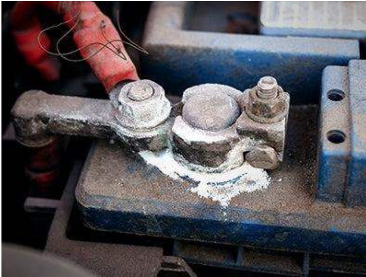
Photo: Battery oxidation
